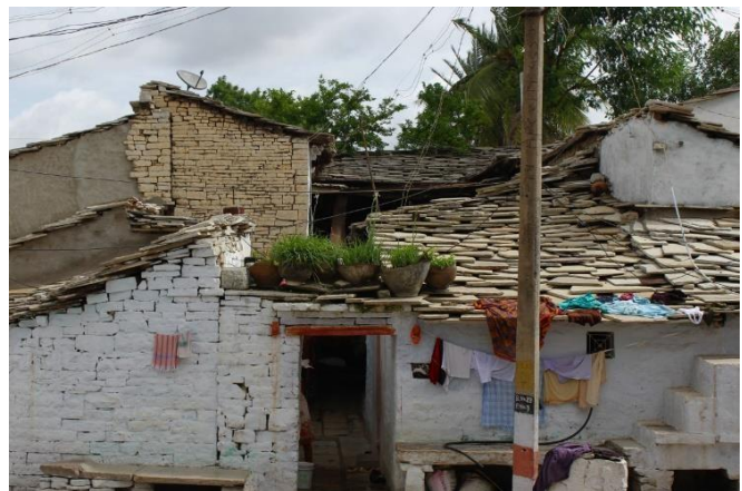
Fig.23. Typical house showcasing Lime stone wall and roof
