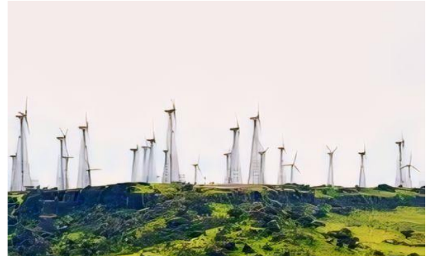
Fig.1.2 Chalakewadi Wind Farm
