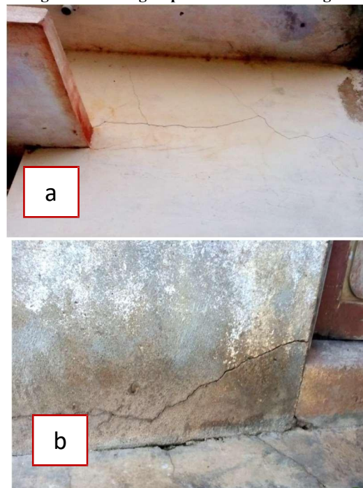
Figure.8 (a) horizontal crack formation near window-(L2) Figure.8(b) horizontal crack formation developed between the ground slab and the external substructure wall
