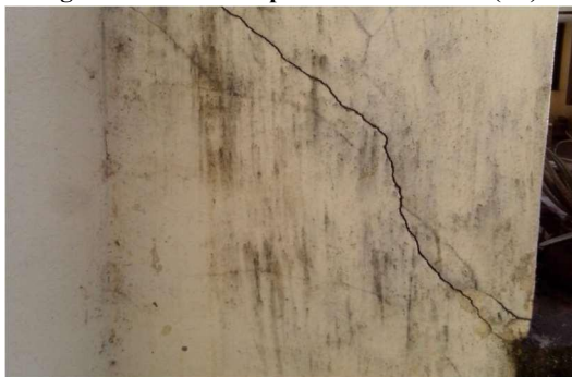
Figure.10 crack developed in external wall (L4)
