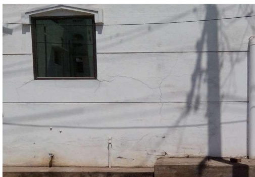
Figure.9 crack developed in external wall (L3)
